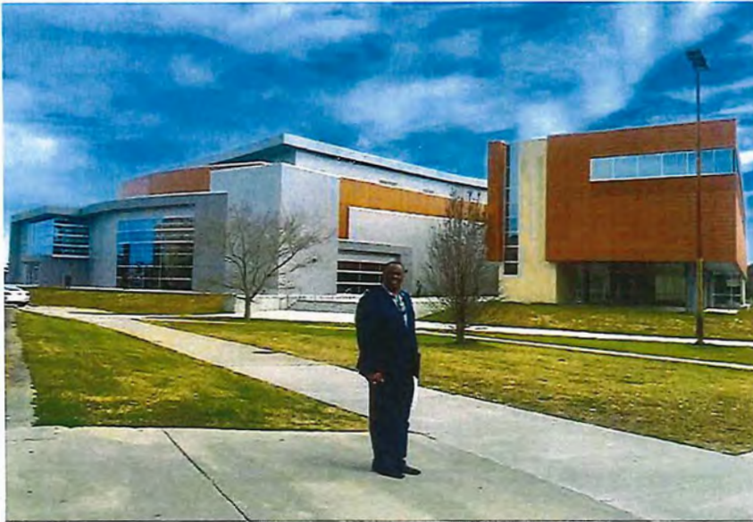
SUNO New Arts and Humanities Building
