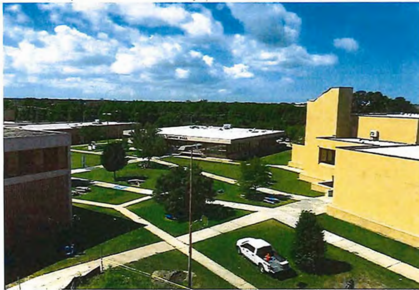
SUNO Re-Roofing projects and sidewalk repairs
