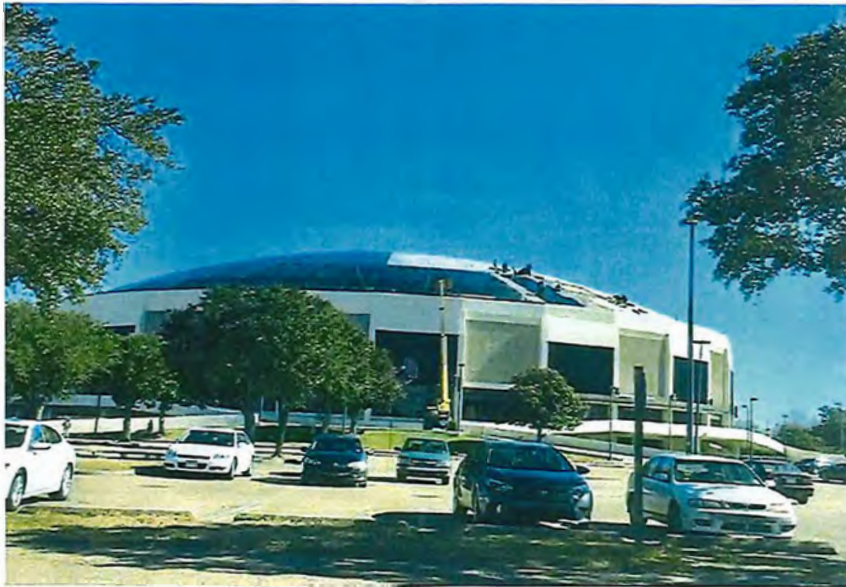
SUBR F. G. Clark Activity Center ADA upgrades and renovations
