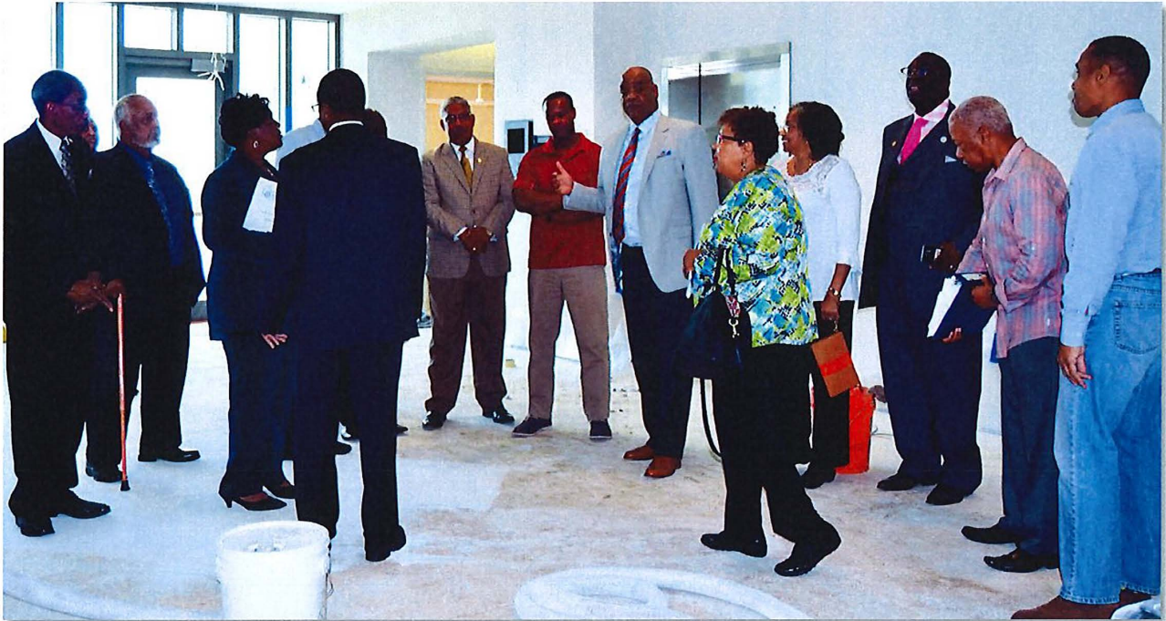
Chancellor Lisa Mims-Devezin, standing third from left, took members of the Southern University System Board of Supervisors, including Board Chair Ann A. Smith, on a tour of the Millie M. Charles School of Social Work Building. Construction of the building is expected to be complete by the end of the year.
