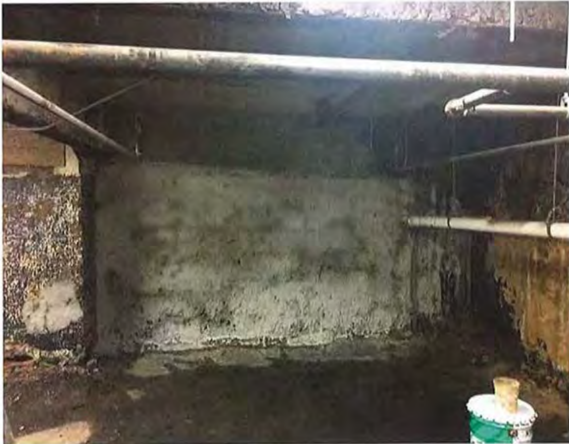
Basement waterproofing in progress
