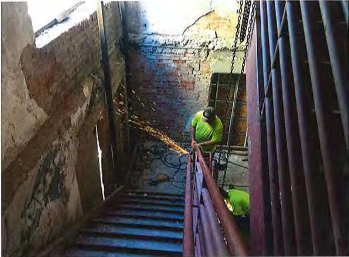
Steel stair framing system in progress
